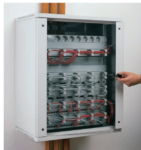
6. Installation is now complete.
