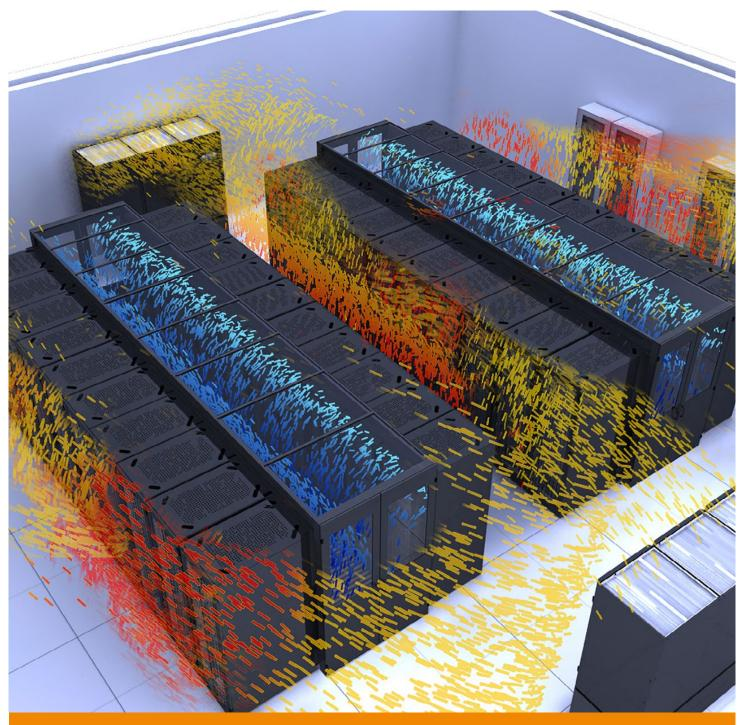
Vertiv<sup>™</sup> SmartAisle<sup>™</sup> containment – systematically separating cold from warm air forms the basis of an energy-efficient data-center
