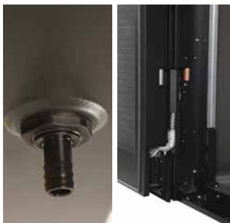
Condensation discharge supports Condensation pan
