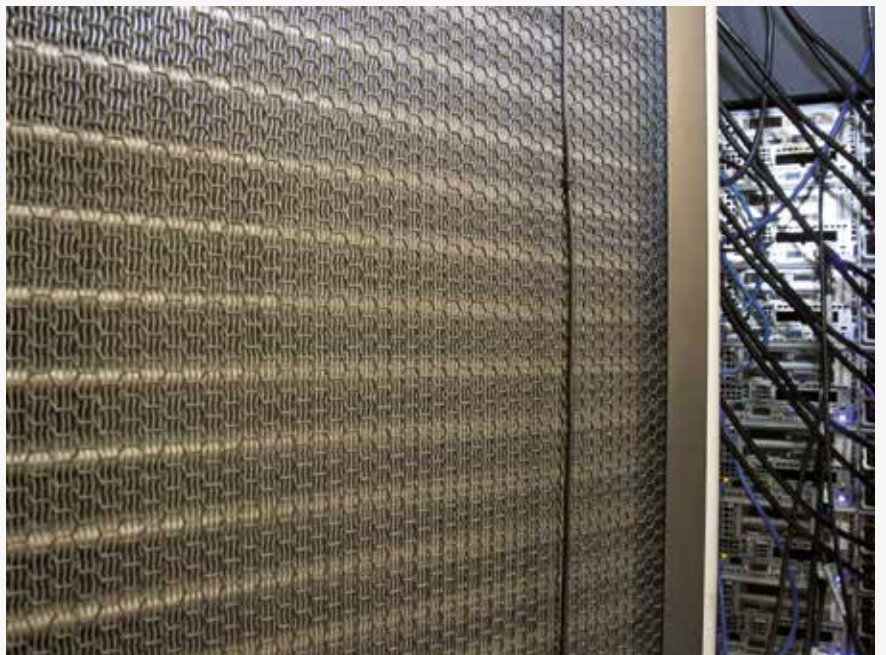
Vertiv Knürr DCD Cooling Door in a server cooling application
